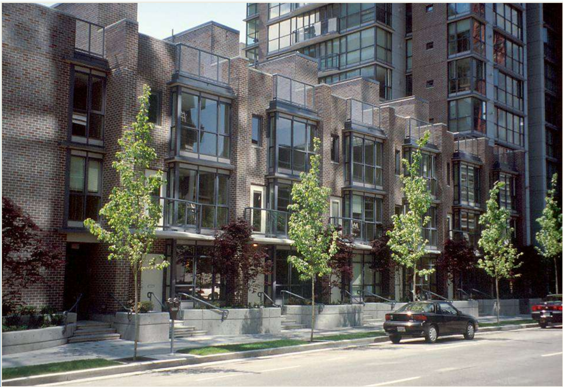
A townhouse podium at base of highrise buildings to create pedestrian-friendly streets
